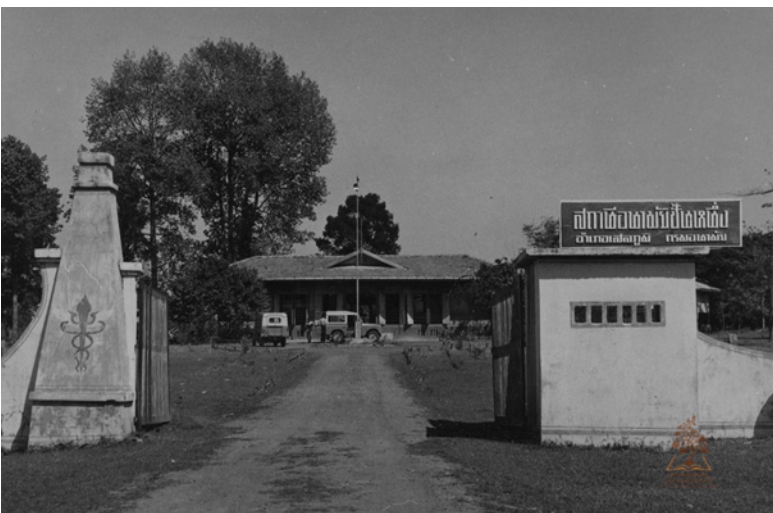
Figure 75 Image of the first-tier Health Center, Selaphum District, Roi Et Province.
