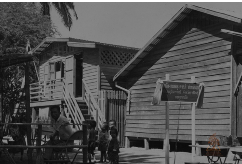
Figure 73 Image of the Midwifery Center, Nakhoo Subdistrict, Kuchinarai District, Kalasin Province.
