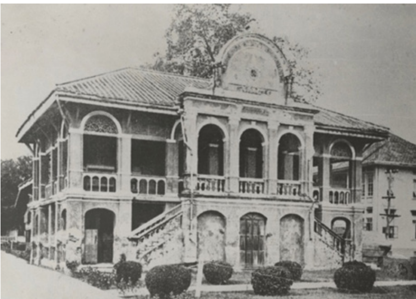
Figure 8 Saovabhark Building used to serve as a special patient ward and dormitory for nursing students.
