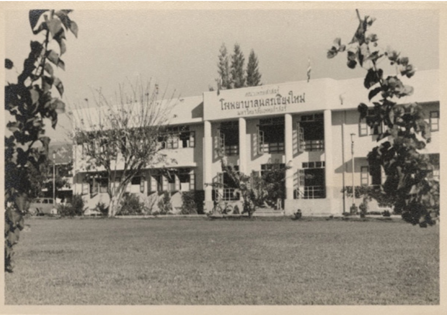
Figure 31 Building Construction at the Faculty of Medicine, Nakhon Chiang Mai Hospital, 1962
