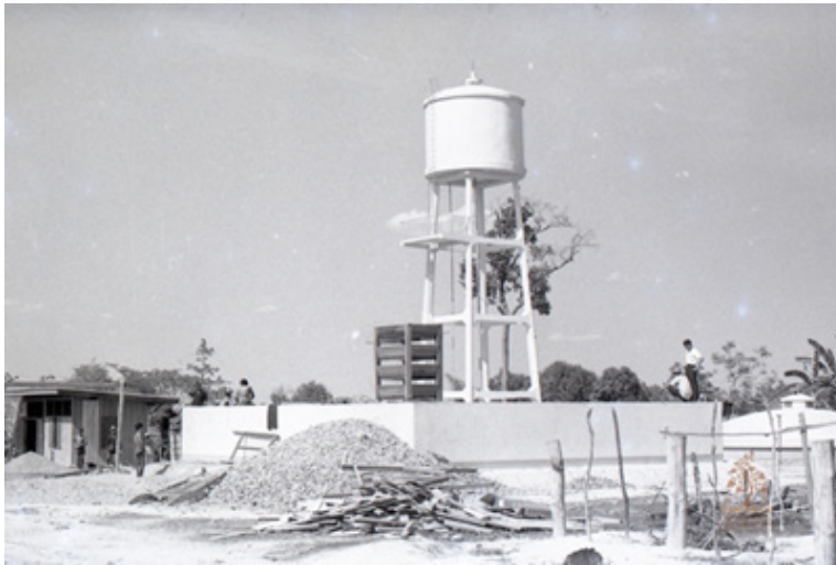
Figure 58 The image of the rural water supply project in Khon Kaen Province, dated 1967.
