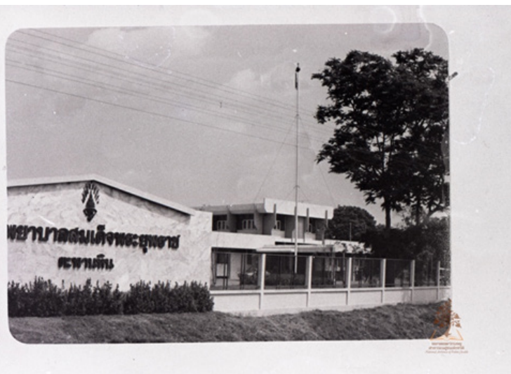
Figure 71 Image of Somdet Phra Yupparat Hospital, Tapan Hin District, Phichit Province
